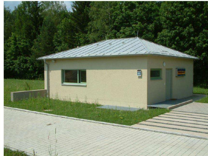
Geothermal district heating station Pullach / Isartal (on the surface)
